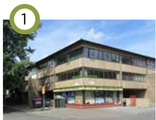
Fishermead 1 and 2 (MKDC, 1972) Three storey houses backing onto landscaped greens. Facades of glazing and fibre cement panels spanning between the party walls. Projecting balconies form carports beneath. Corner blocks of flats and maisonettes with the ground floors either fitted out for commercial use or left vacant for such uses in the future.
