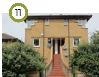
Oldbrook 6 (MKDC, 1982) Shared ownership scheme with standalone blocks comprising two ground floor flats and sweeping staircase to the two maisonettes on the first and second floors, a development of the blocks in Oldbrook 1 and a clever way to give architectural dignity to small dwellings.
