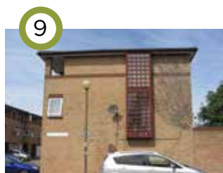
Oldbrook 2 (Colquhoun and Miller, 1980-83) Three storey mews courts leading towards CMK with two storey cross streets with linking pergolas over the parking spaces. Oriol staircase windows form dramatic features at the ends of the taller blocks. Crinkle crinkle walls line the interior greens.
