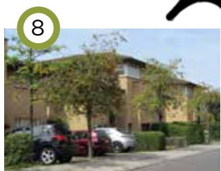
Oldbrook 1 (MKDC, 1980) Three storeys and pitched roofs from the outset. Backing onto the Local Park, cluster blocks combining smaller units to make detached pavilions – a new departure for MKDC. Shallow pitched roofs and deep eaves in the manner of Frank Lloyd Wright's Prairie Houses.
