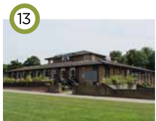
The Cricketers Public House and Meeting Place (David Byrne Associates 1982-3) Broad hipped roofs with a pop-up manager's flat. The original brightly coloured timberwork has suffered in a subsequent redecoration. Enjoyable interior stained glass on a cricketing theme by Brian Milne.
