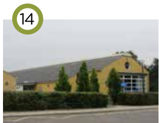
Oldbrook First School (Bucks County Council, 1994) One of a new wave of school designs that moved away from the more traditional image adopted by BCC. Linear design with classrooms off a spine. Big gridded window overlooking Oldbrook Green. Subsequent extension by Stenton Obhi Architects.
