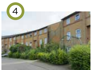
Fishermead 7 (MKDC, 1982) Three storey crescent that was originally planned for a mirror site in Conniburrow but moved to Fishermead as a result of poor ground conditions. A suitably grand scheme to mark the termination of MKDC's rental housing programme.
